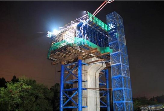
Casting of support #0 in the night, 8/28/2019
