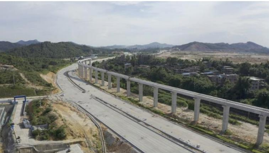
1st construction phase in 2021
