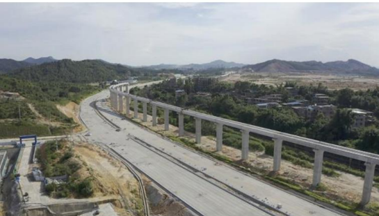
1st construction phase in 2021
